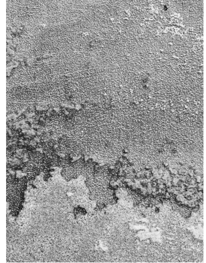
Salt 9802 (Efflorescence)
